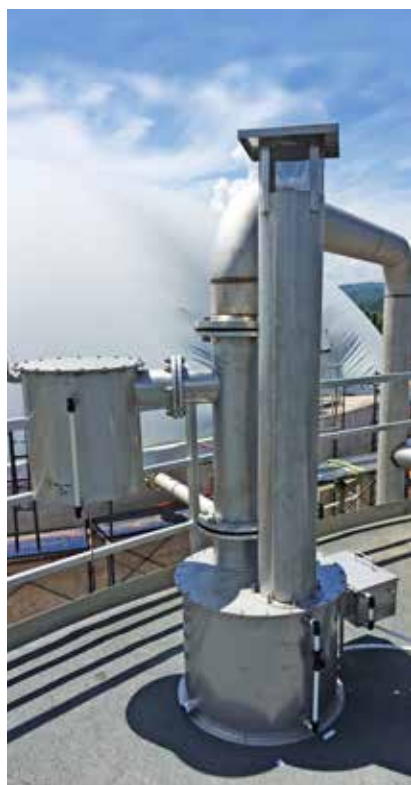
HYDRAULIC SAFETY VALVE WITH ANTI-VACUUM
