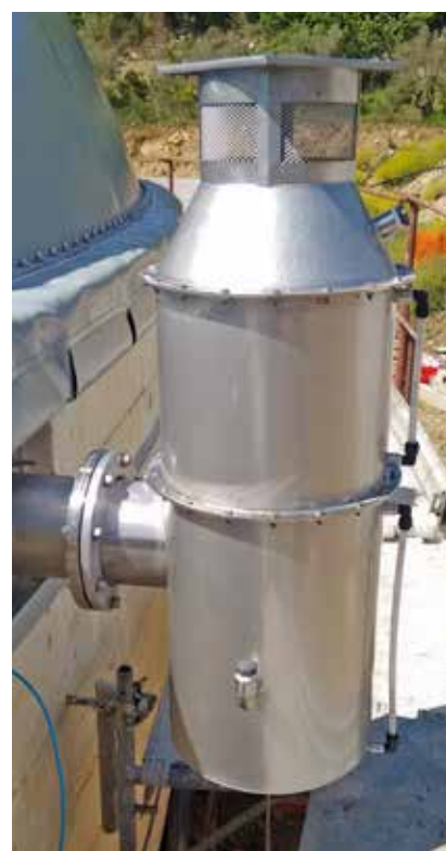
OVERPRESSURE AND ANTI-VACUUM SAFETY VALVE
